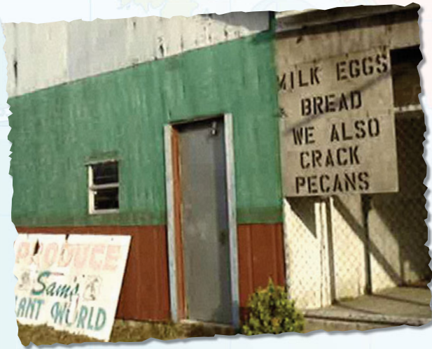
People do whatever they can to survive. This enterprising proprietor uses the building for an unusual combination of purposes: a "plant world," along with the sale of milk, eggs, bread, and, in a quaint southern touch, cracking pecans.
