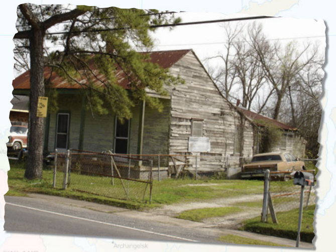
With little work available, it is difficult to afford adequate housing. This house, although cobbled together and in disrepair, is a family's residence.
